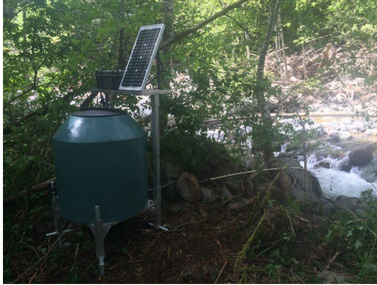
Figure 2: A typical AutoSalt installation showing Control Box, 300L Brine Tank, custom stand, and injection pipe.
